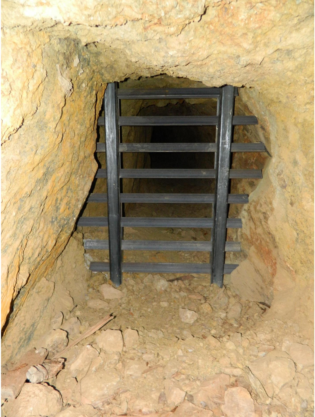
New gate installed on Catalina to protect bats. Photo by Julie King
